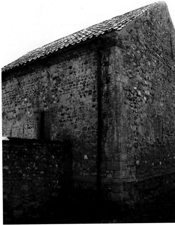
Fig 16 A farm building in Little Walsingham with a quoin built entirely of recycled medieval freestone. Photograph, J. Thorpe, 2016
