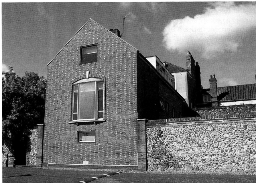
Fig 21 House in Norwich Cathedral Close, post second world war, using Flemish bond with the headers replaced by individual flints. Photograph, J. Thorpe, 2016
